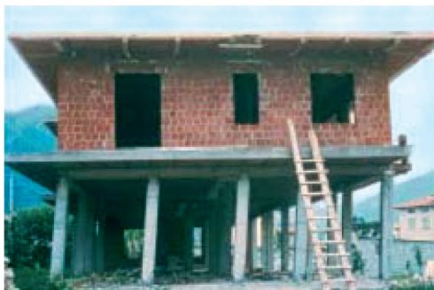
4/1 This sway mechanism in the ground floor of a building under construction almost provoked a collapse (Friaul, Italy 1976).
