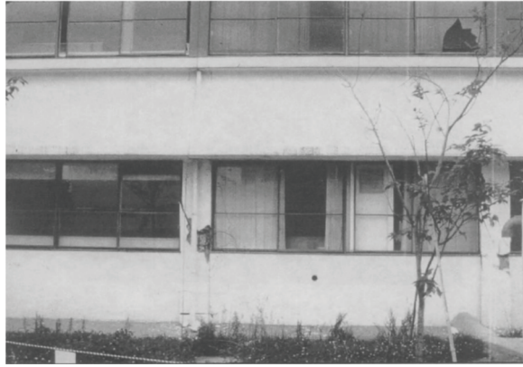
Figure 3-35 Captive Column Failure, Japan, Miyagi-ken-oki, 1978
