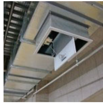
Figure 4-12 Smoke Exhaust
