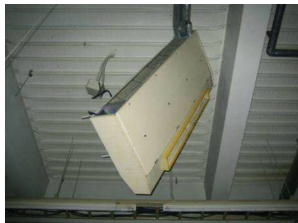
Figure 4-23: Example of Breakage of Suspension by Earthquake
