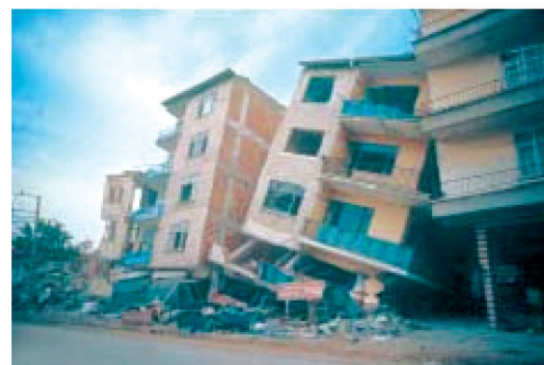
4/2 Sway mechanisms are often inevitable with soft storey ground floors (Izmit, Turkey 1999).
