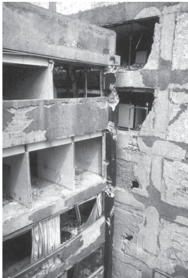
Figure 3-39 Damage caused by Hammering of Adjacent Buildings due to Inadequate Separation in 1985 Mexico Earthquake [Reference: Design of Concrete Structure, 14th Edition by Arthur H. Nilson]
