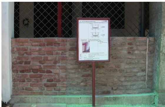
Figure 3-37 Slit for the Prevention of Shear Fracture
