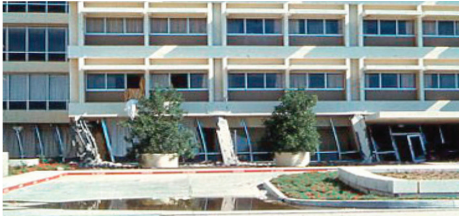
Figure 3-21 Olive View Hospital, San Fernando Earthquake, 1971, showing the extreme deformation of the columns above the plaza level.
