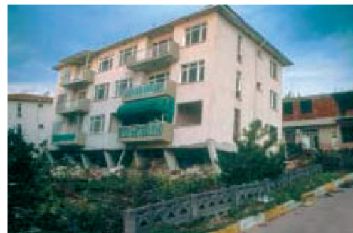
4/3 Here the front columns are inclined in their weaker direction, the rear columns have failed completely (Izmit, Turkey 1999).
