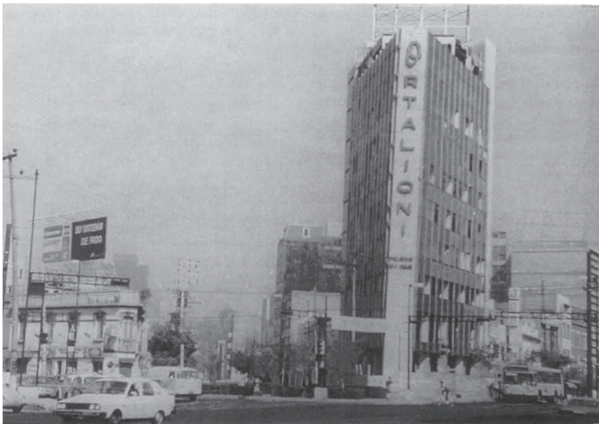
Figure 3-18 Distortion in Wedge Shaped Building, Mexico City, 1985
