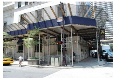
Safety canopy with curb board
