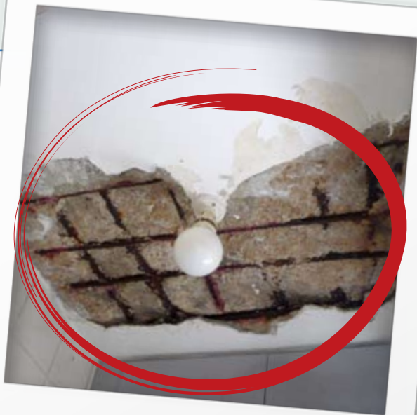
Spalling of concrete at ceiling
