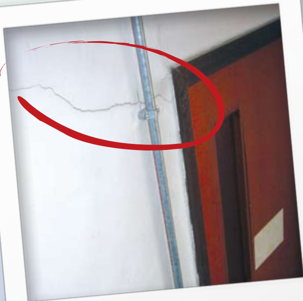
Cracks at the corner of door frame
