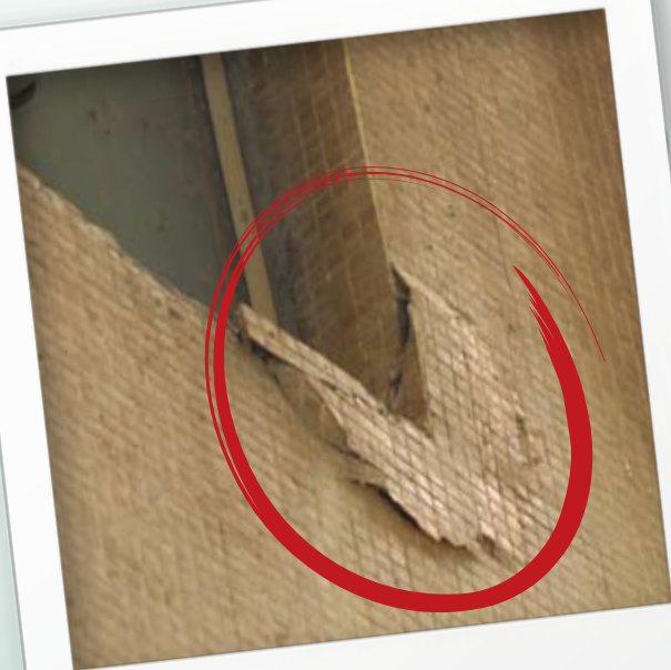
Bulging and loosening of wall tiles
