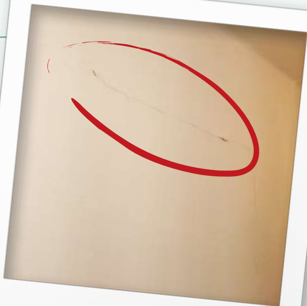
Fine cracks on wall
