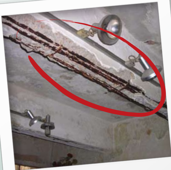
Spalling of concrete at beam soffit
