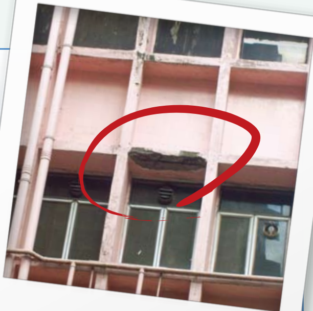
Defective architectural fin
