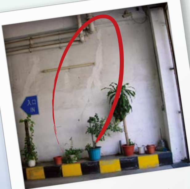
Cracks on partition wall
