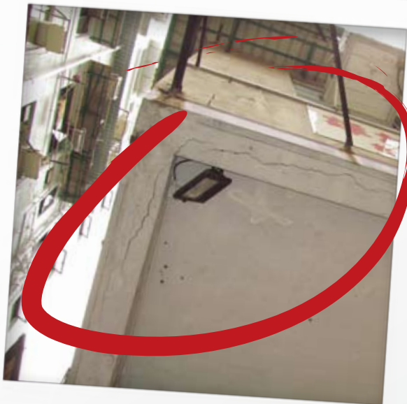
Cracks on the beam
