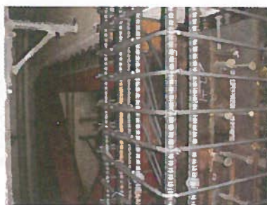
(l) RC wall and steel framed bracing
