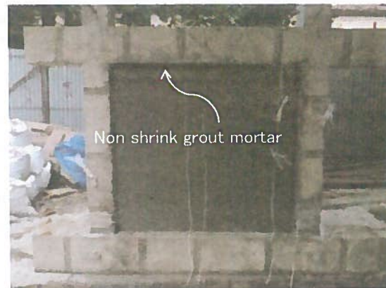
(b) Non-shrink grout mortar work done at the top of wall portion
