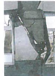
短柱のRC柱の剪断破壊 (Shear failure of short column)
