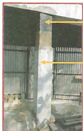
Method 5: Carbon fiber wrapping
