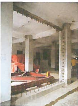
(1) Chemical anchor at beam and column
