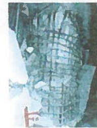
2階のRC柱の剪断破壊 (Shear failure of 2nd storey column)
