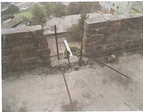
(i) Sampling of re-bar for tensile test
