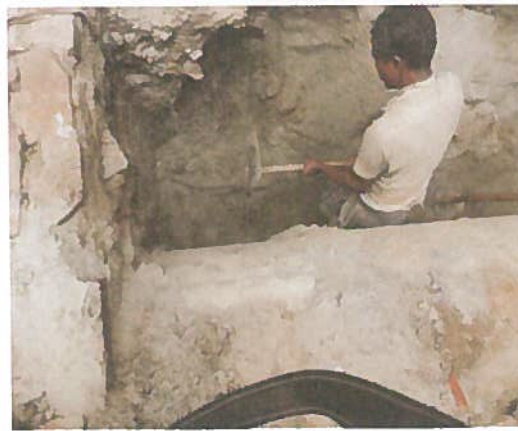
(j) Exposure of foundation (Note: wearing helmet is suggested)
