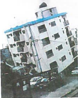
集合住宅1階の崩壊 (Collapse of roof in 1st storey building)
