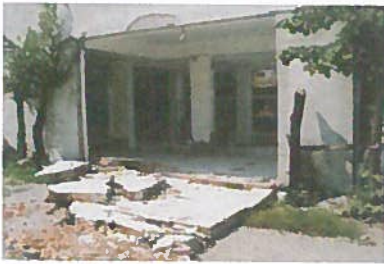
Overturning of brick infill wall
