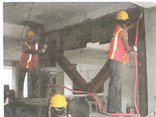
(f) Pressured non-shrink mortar grouting at the top in progress
