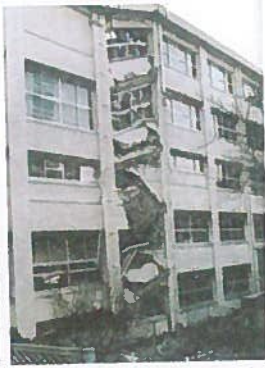
1階の崩壊 (First storey collapse of three storey)
