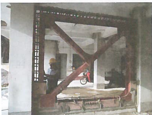
(e) Erected steel framed brace
