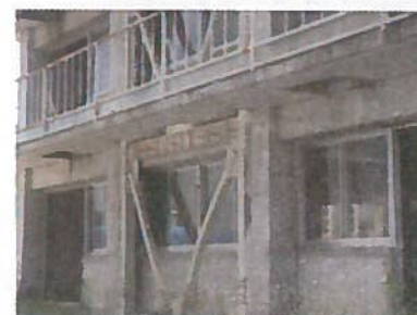
(m) Steel framed brace of a school building, at E-defense, Hyogo
