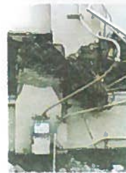
剪断時のRC柱の剪断破壊 (Shear failure of column with aggregate)
