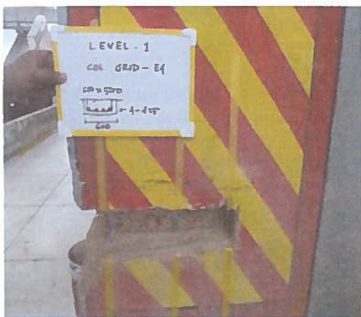
(c) Exposure of re-bar
