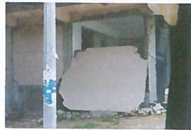
Failure of infill brick wall
