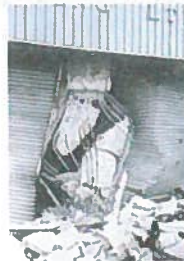
RC柱の剪断破壊 (Shear failure of column with widely spaced shear reinforcement)
