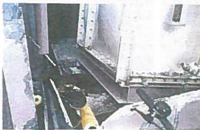
Sliding of water tank
