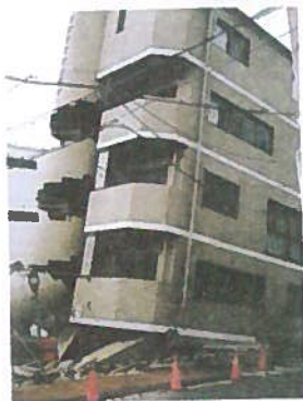
1階の崩壊 (Storey collapse at 1st floor)
