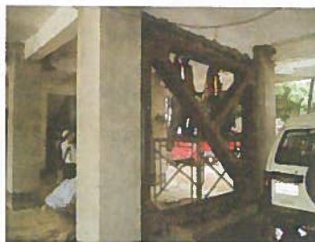
(3) Erection work of steel framed brace
