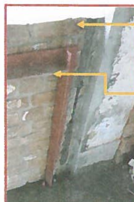
Method 6: Seismic slit on brick standing wall
