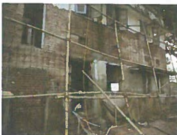
(1) Re-bar work of perimeter brick wall
