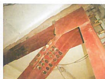
(4) Connection of steel framed brace
