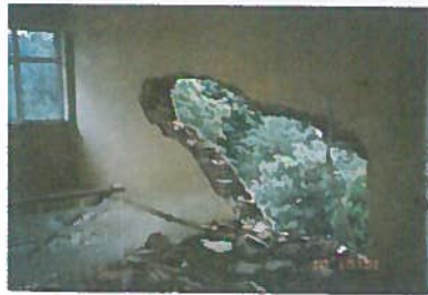
Drop of infill brick wall
