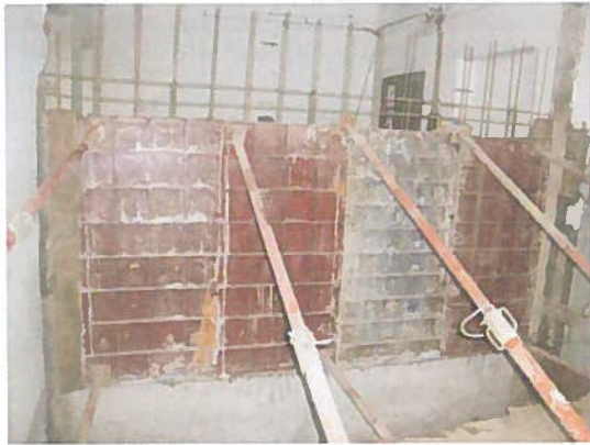
(a) Re-bar and concreting work
