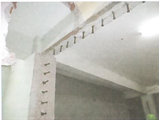
(c) Post installed anchor work
