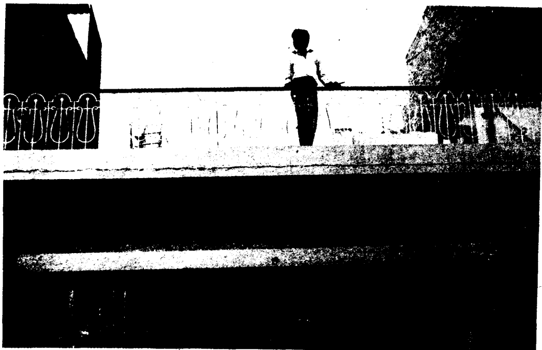
Photo 3 Horizontal Crack at the Support of a Brick-cum-Iron Railing Over an RCC Cantilevered Roof Slab due to Different Shrinkage and thermal Movement
