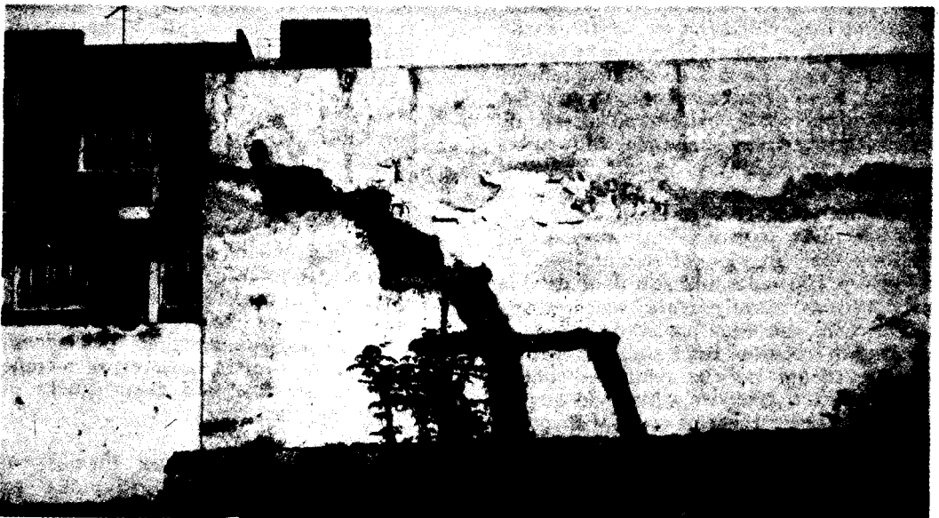
Photo 12 Diagonal crack in the corner of a building due to foundation settlement; crack has been repaired by providing RCC stitching blocks
