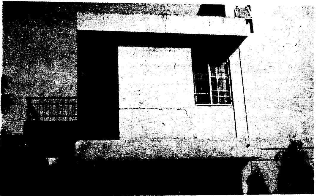
Photo 7 Horizontal Crack in Masonry Supported on a Cantilevered Canopy Slab due to Elastic Deformation, Shrinkage and Crack in RCC Canopy Slab
