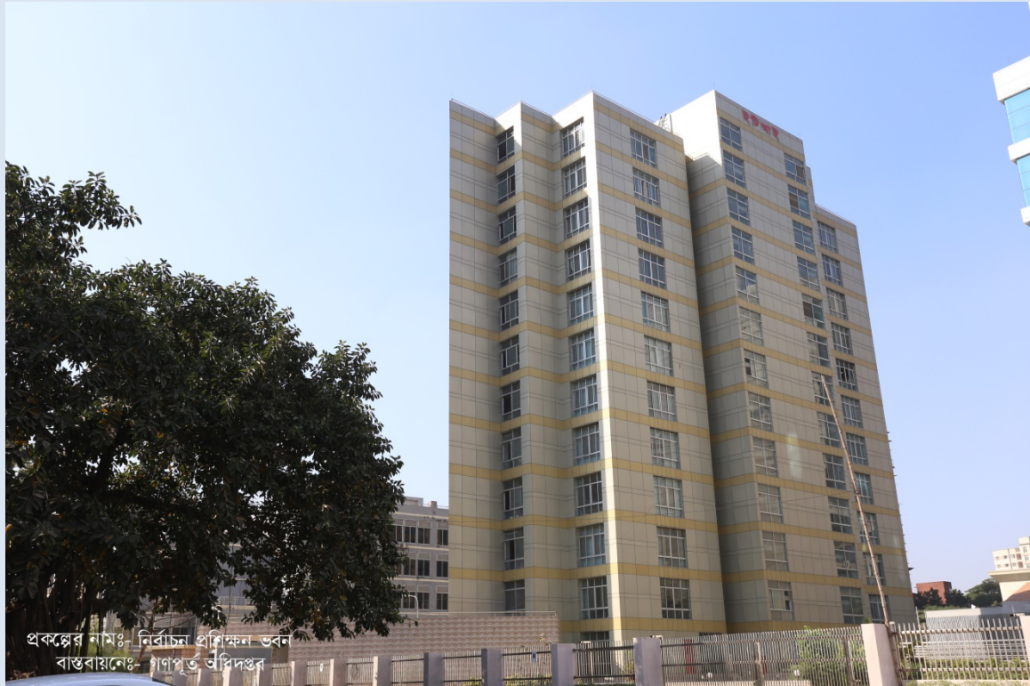
Construction of Election Resource Training Center
