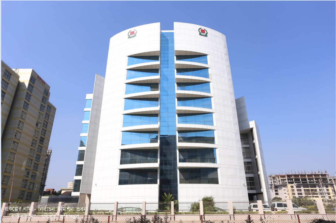
Construction of Election Resource Center
